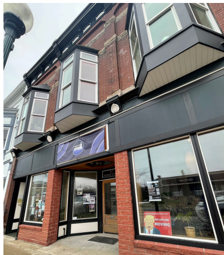
Street view of the North Coast Works Building, 417 Howard Street.
